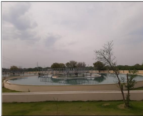
Fig. 4. View of the Clari-flocculator
