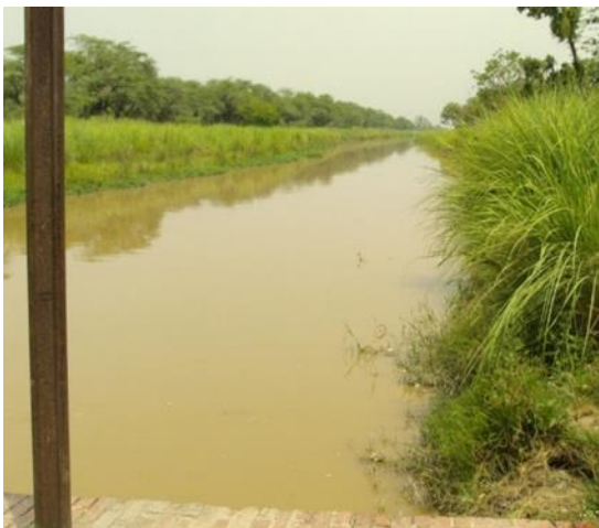
Fig. 1. View of the Ganga Canal at Palra, District Bulandshahr
