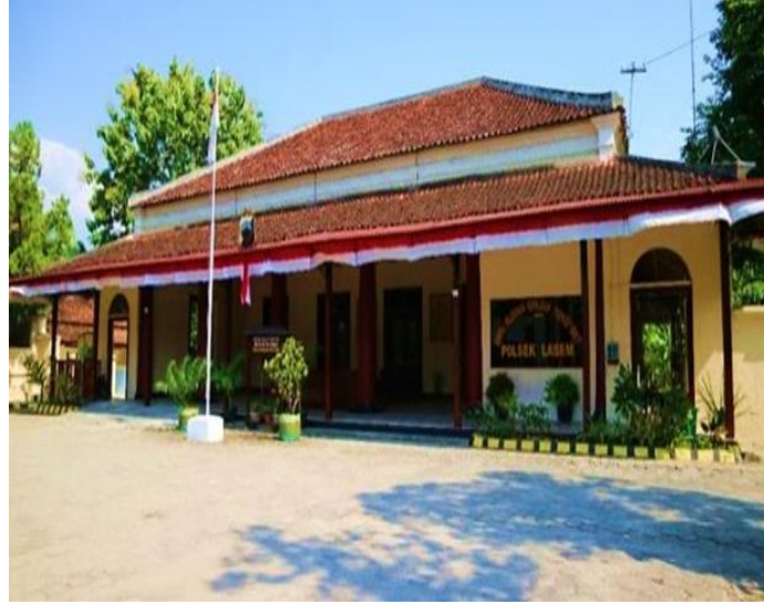
Figure 13. Lasem District Police Office Source: Putranto dan Pradnyawan, 2018
