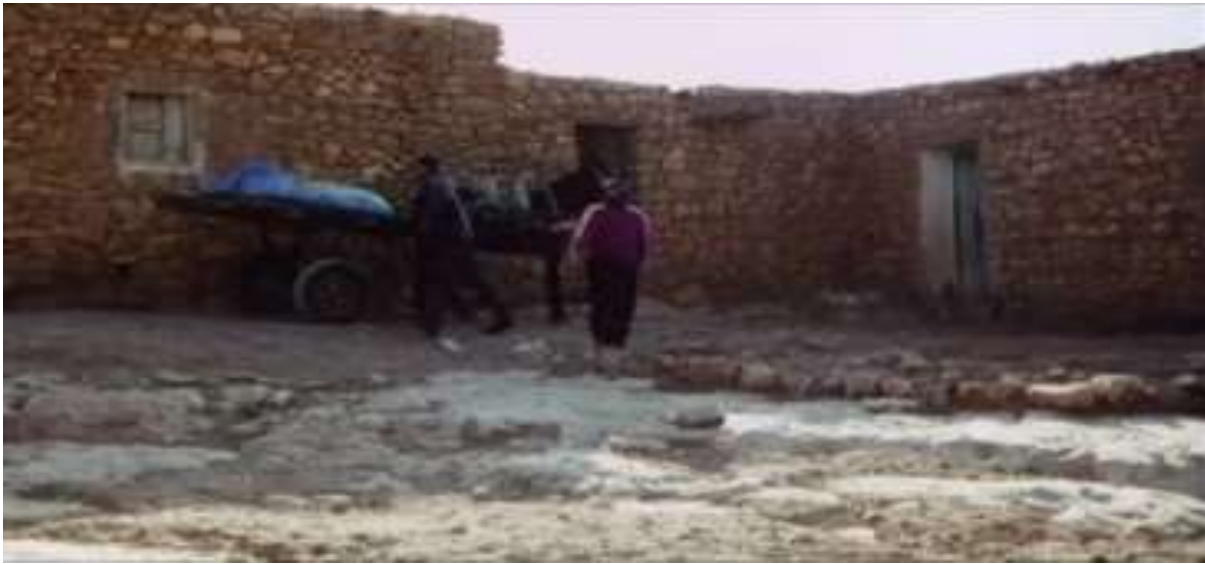
Figure 12: Rural housing conditions. (36:57)
