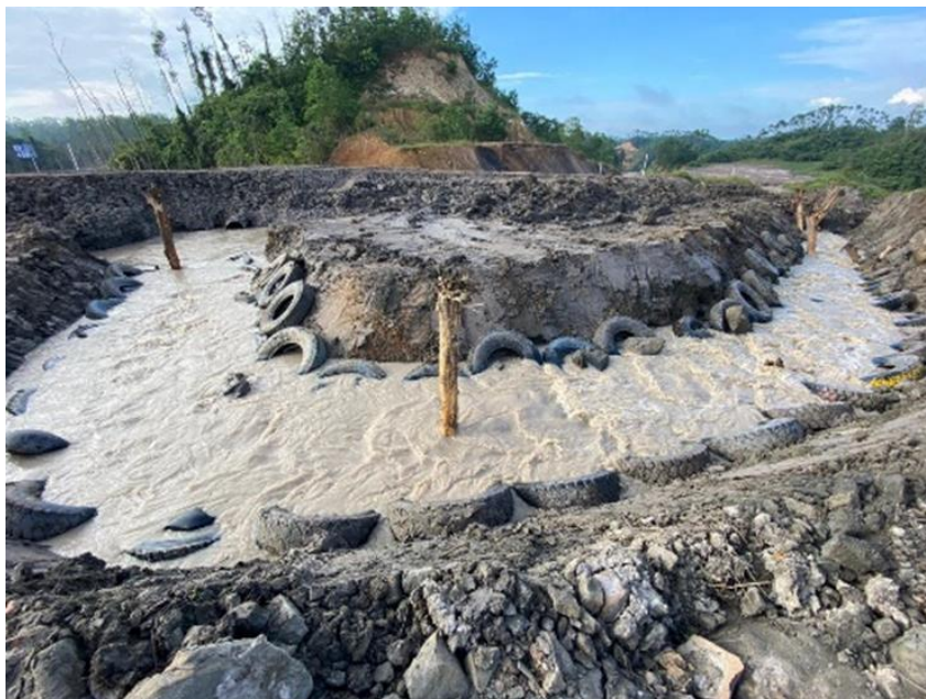
Figure 1. Tyre Drop Structure
