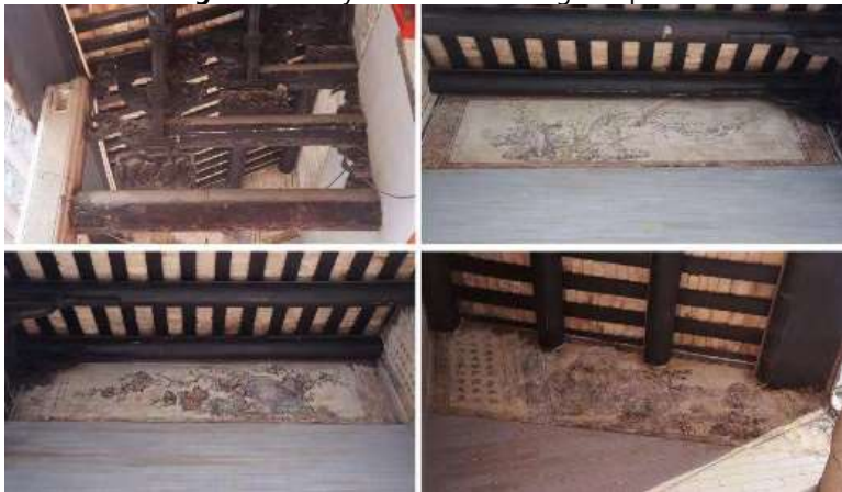
Fig.37. The woodcarving beam frame and wall frieze of the head gate of the Sanwang Temple
