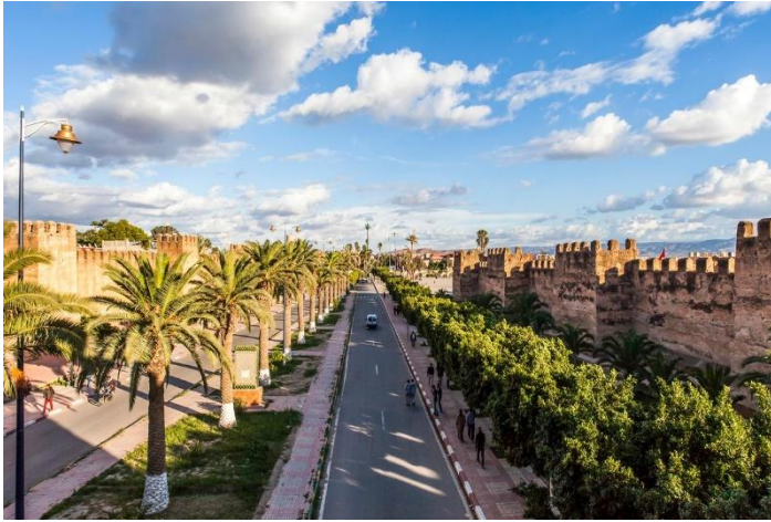
Fig.1: The wall of Taroudant. Photo credit: Google.
